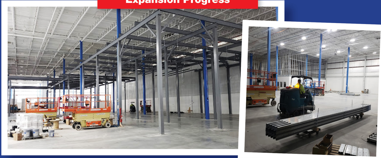
DUE TO BE COMPLETED 2ND QUARTER 2022
