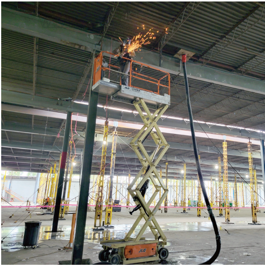
A worker cuts a section of the roof at Unitex's new Hartford warehouse, at 121 Wawarme Ave. The roof is being raised by 10 feet.
